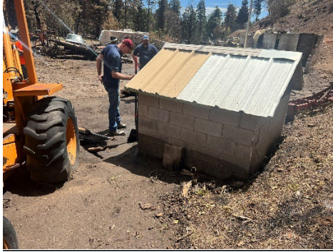
Figure 1. Cedar Creek, Ruidoso, one week after the Blue 2 fire. Heavy sediment loads partially buried a wellhead with debris. The backhoe is maneuverable on the road. (Photo courtesy of SMA Engineering)
