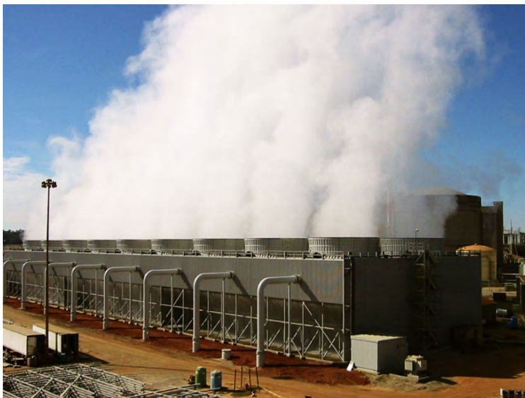
Fig. 2. Example plumes rising from a 10-unit mechanical draft cooling tower. [11]
